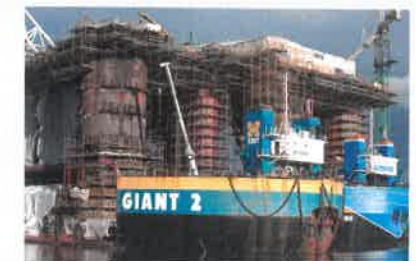
► An oilrig under construction
