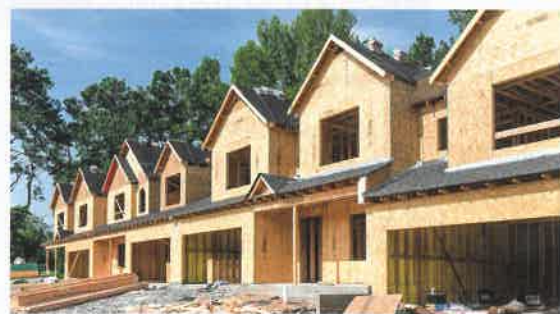
▲ Construction of new houses can be slow
