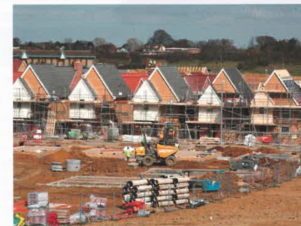
▲ Construction at a building site
