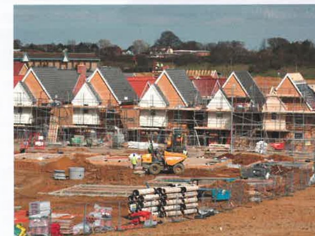
▲ Construction at a building site
