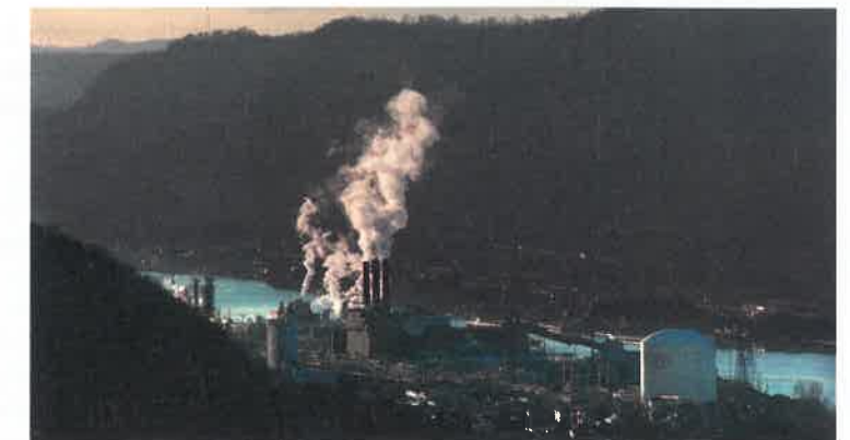
▲ DuPont's Belle plant, Kanawha County, West Virginia, USA
